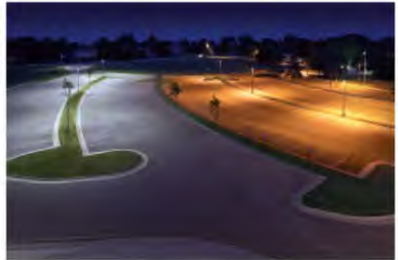
Comparison of LED fixtures (left) versus High Pressure Sodium (HPS) fixtures (right)
